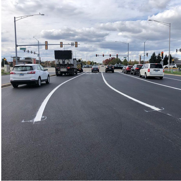
New asphalt surface and permanent pavement markings
